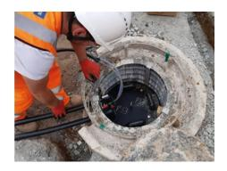
The patented Hiperpile utilises the high thermal capacity of a water-filled void to store thermal energy in the short term. This enables the foundation itself to provide extremely high, short-term peak loads whilst also meeting annual base load demands.
